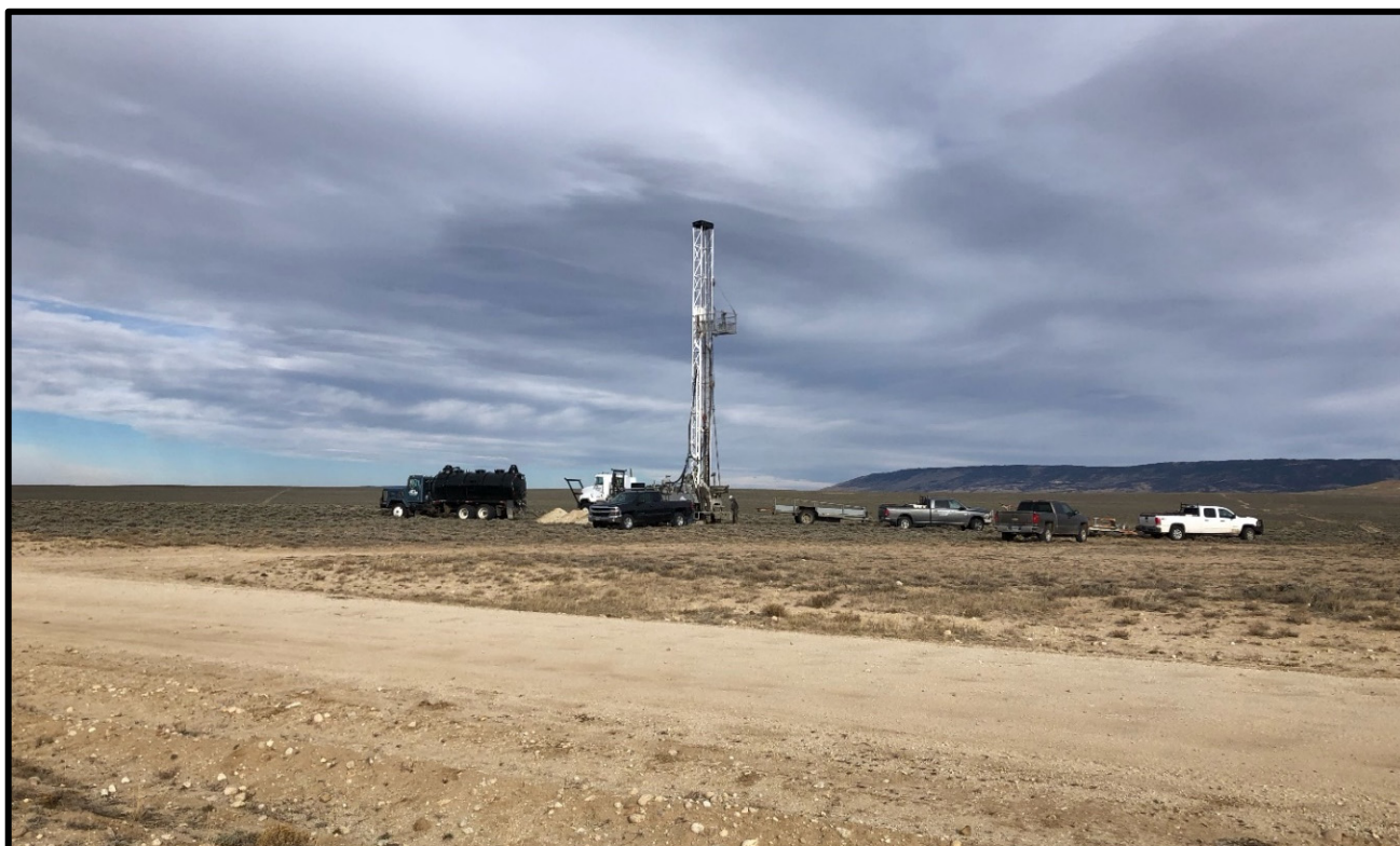
FIGURE 5: MUD ROTATRY DRILL RIG OPERATING, ODIN ISR URANIUM PROSPECT, GDB WYOMING, USA
